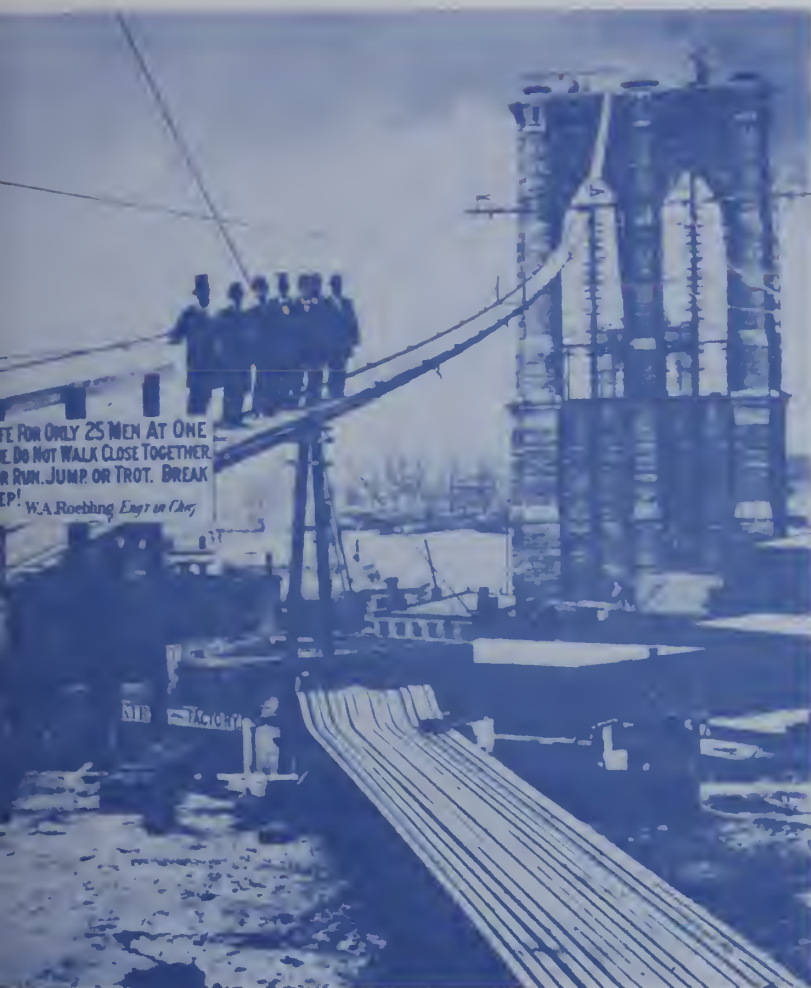
Footwalk to the tower, with steel anchor bars in foreground which linked the cable strands in each anchorage to four 23-ton cast iron plates, one for each cable.
